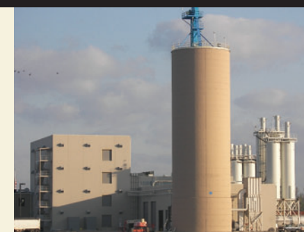
SEMO Milling, a founding partner of MOR, operates a food-grade corn mill in Southeast Missouri (pictured above) which houses the MOR-Frac™ pilot fractionation system
